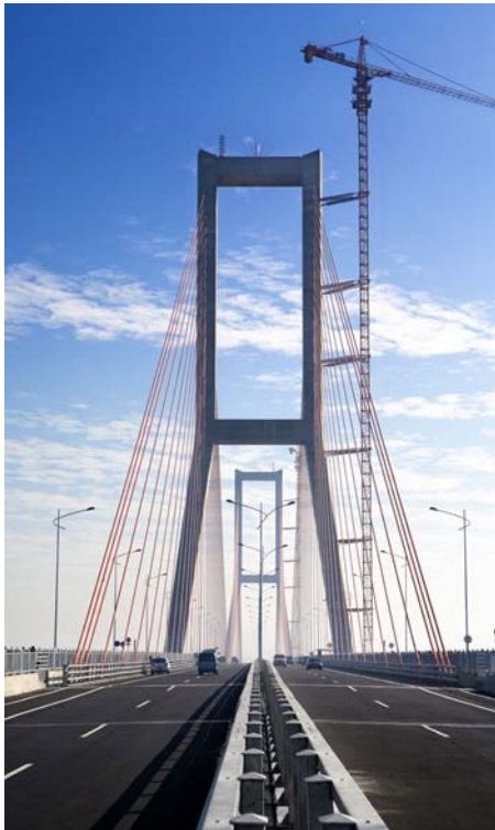
SuraMadu Bridge, Indonesia
